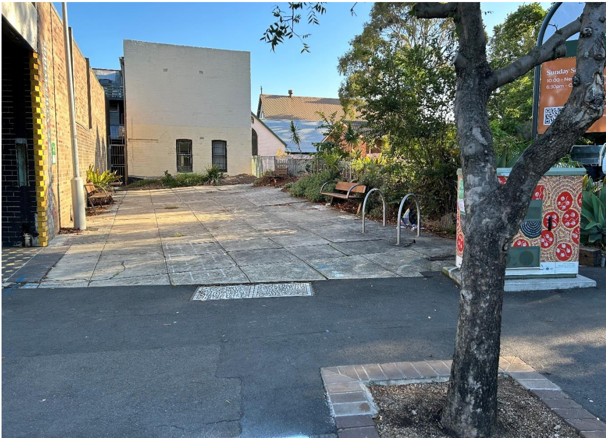
Existing reserve looking south towards the rear of the site– the paving is at the end of its lifecycle. The site is exposed from the recently removed neighbouring trees. Small planting area in poor condition.
